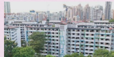
View of Block 2 at Jalan Bukit Ho Swee.
