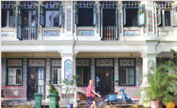
Pre-war terrace houses along Petain Road.
