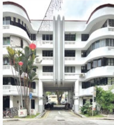
Five-storey flats at Moh Guan Terrace.
