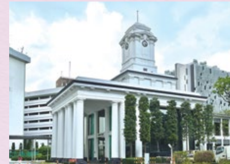
Singapore General Hospital at Outram Road.
