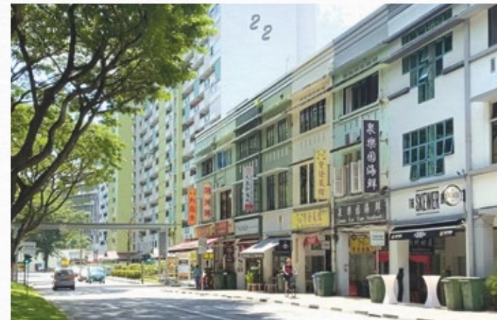
Block 22 Havelock Road stands next to old shophouses.
