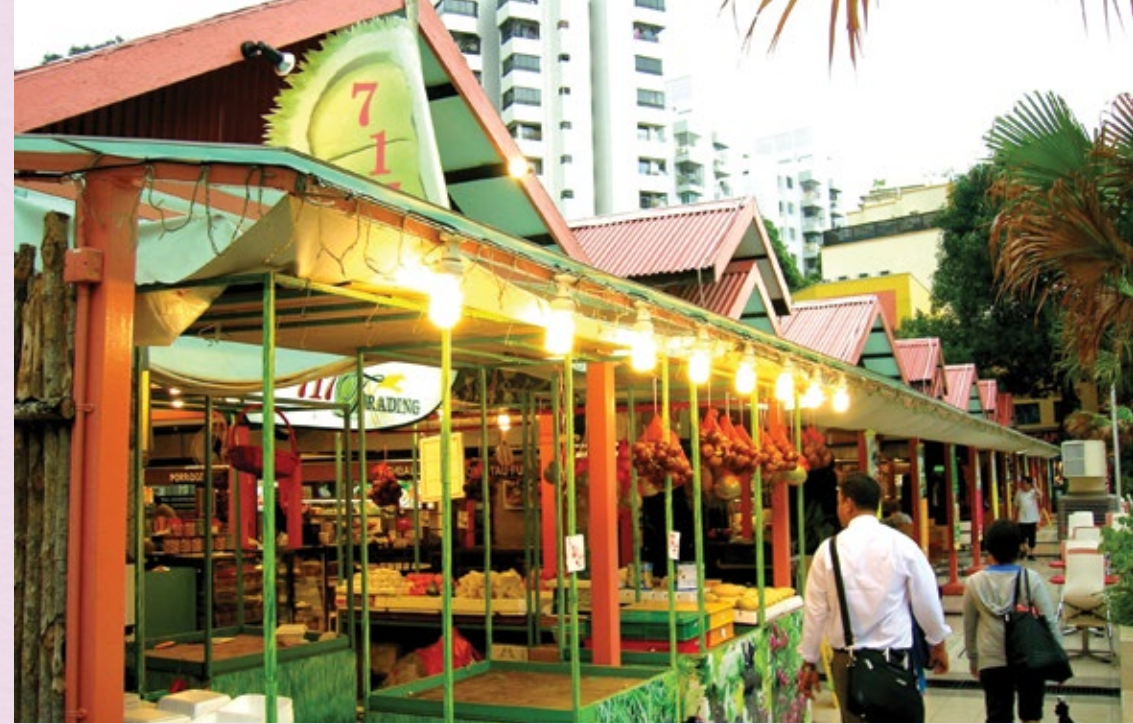
Balestier Market and Food Centre at 411 Balestier Road is more than 100 years old.
