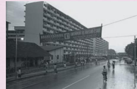
Former HDB flats at Cantonment Road.
