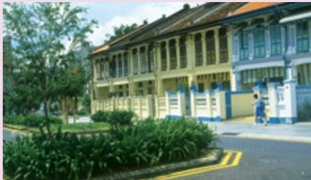
Conserved houses at Emerald Hill.
