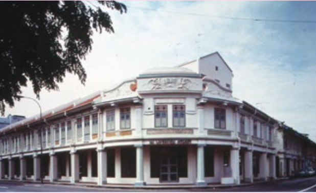
Shophouses at Jalan Besar.
